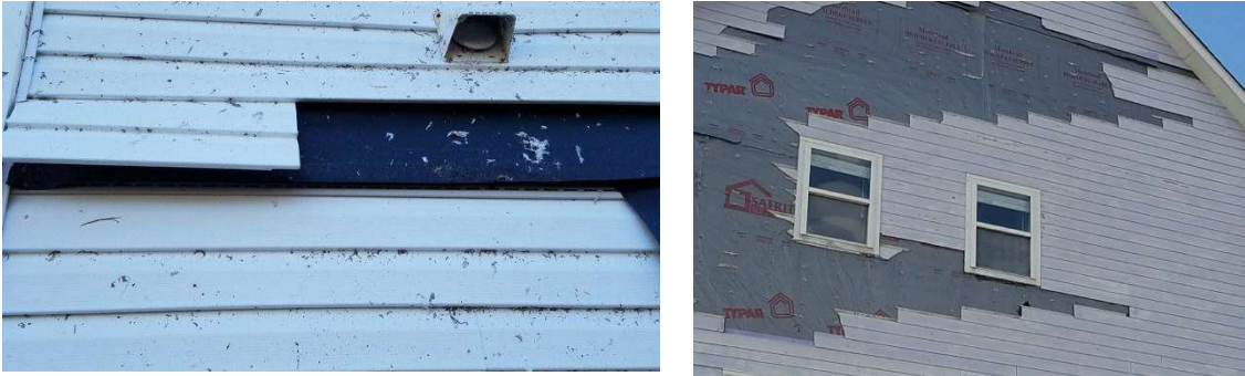
Figure 13. (Left) Vinyl siding indicated by “double” slats; (right) non-vinyl product indicated by “single” slats and lack of perforated nailer hem.
