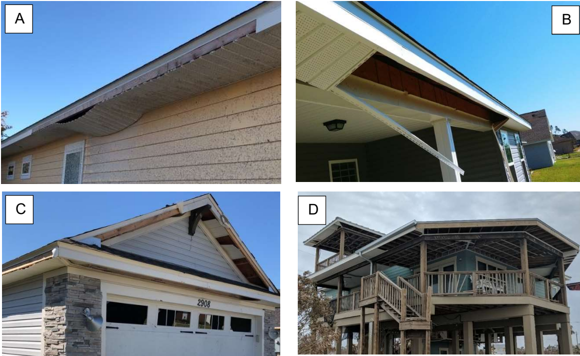
Figure 25. Soffit and fascia damage. (A) a 2017 home in Beacon Hill subdivision; (B) soffit damage without corresponding fascia damage to a 2015 home in Cedar's Crossing neighborhood; (C) extensive soffit and fascia damage to a 2016 home in Cedar's Crossing neighborhood; (D) extensive soffit and fascia damage to a 2012 home seaward of the Coastal Construction Control line in Mexico Beach, FL. Note the lack of fascia failure where the gutter is installed.
