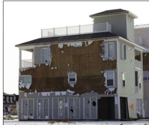
Extensive lost of vinyl siding and housewrap event though high wind panel was used (FEMA 2005)
