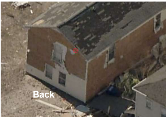
Figure 14. Illustration of damage ratios assigned to each wall surface for a home in Port St. Joe (Bay County) built in 1999.
