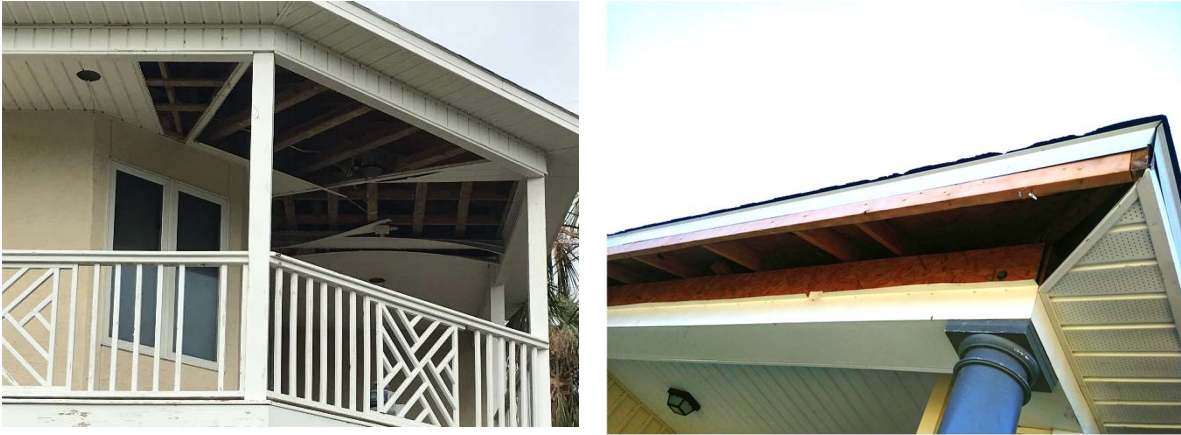
Figure 15. (Left) Failed vinyl soffit on the second story of a 1998 home in the Gulf Aire neighborhood due to Hurricane Michael; and (right) Failed fascia on a 2015 home in the Cedar's Crossing neighborhood due to Hurricane Michael.
