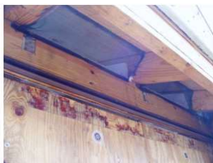
Specimen 4 -The perforated vinyl soffit in conjunction with an insect screen across the threshold of the attic and soffit space
