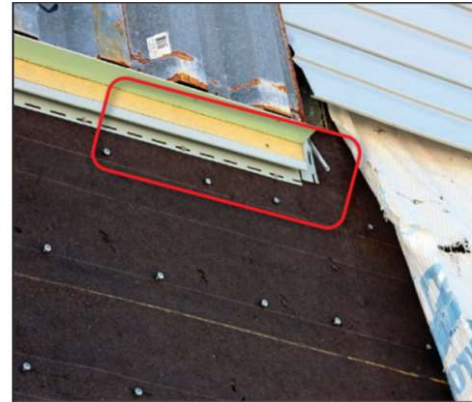
Vinyl siding failure because to lack utility trim under the windows (Fema 2018)
