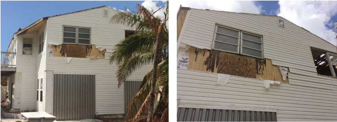
Figure 21. Case Study #2: Failure of a vinyl siding system on a 1958 home on Sugarloaf Key. The vinyl siding was installed in 2004 per the county permit records.
