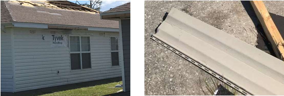
Figure 20. Case Study #1: Minor failure of a vinyl siding system on a 2006 home in the Cedar's Crossing neighborhood for which the siding manufacturer and Miami-Dade Notice of Approval were able to be traced.
