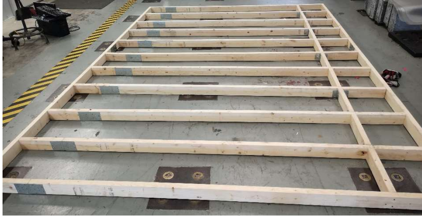
Figure 35. Wood Wall Frame with stud splicing and wood blocking
